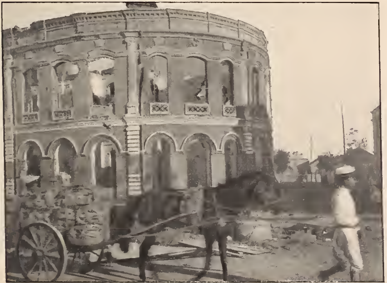
RAILWAY ADMINISTRATION BUILDING, TIENSIN, SHOWING EFFECT OF SHELL FIRE.
